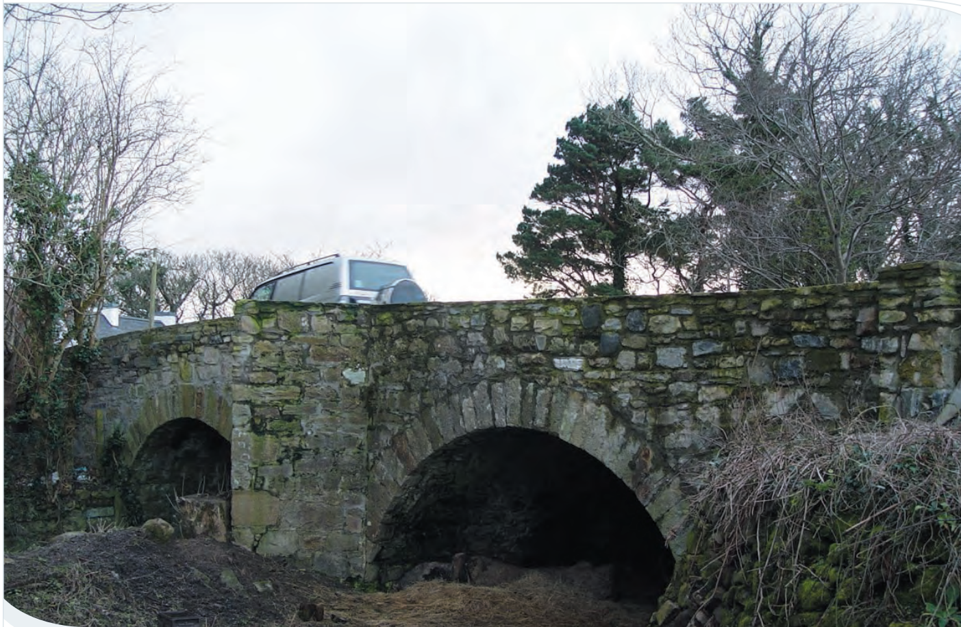
Gortnaderry Bridge after restoration
